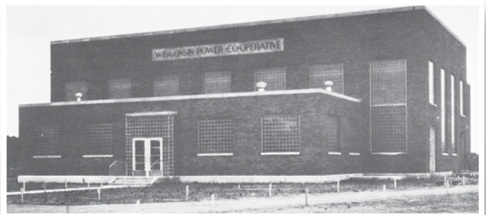
Wisconsin Power Cooperative, which generated the power supplied to Clark Electric's first section of line in 1938, was the first generating cooperative in the nation.
